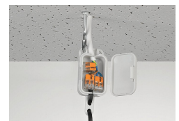
Pendant light connection in a suspended ceiling
